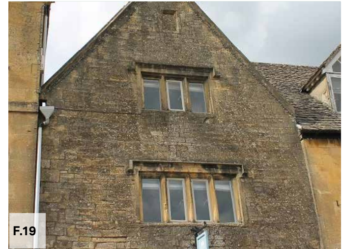
Figure 19: Mullioned windows, High Street
