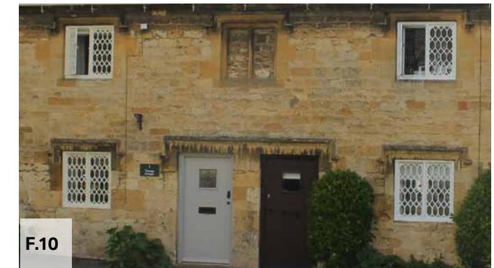
Figure 10: Casement windows, Leysbourne
