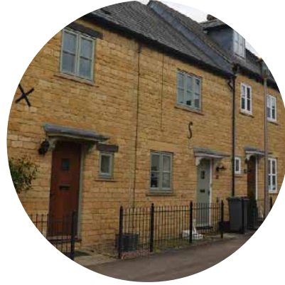
Door hoods and flush casement windows, use of decorative wall plates
