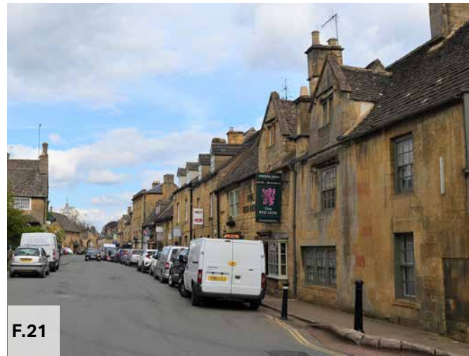
Figure 21: Varied rooflines, High Street
