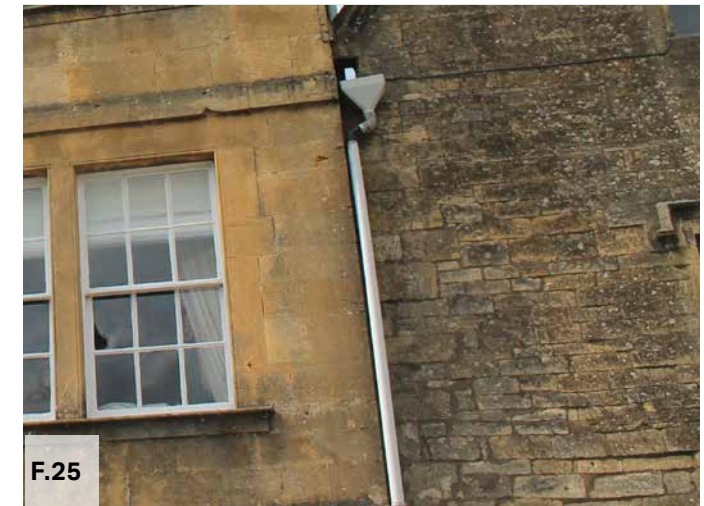
Figure 25: Rainwater goods, High Street
