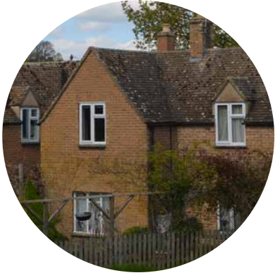
Brick wall material
