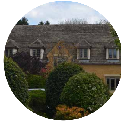
Multiple dormer windows
