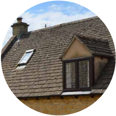
Graduated stone slate roof with rendered dormer window
