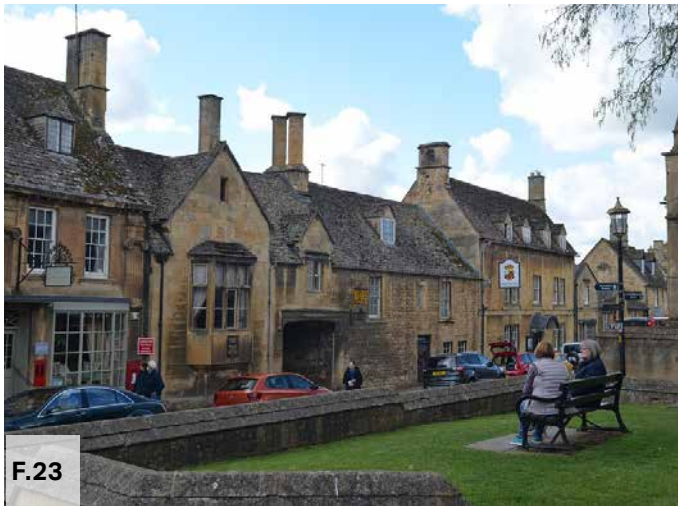
Figure 23: Dormer windows, High Street
