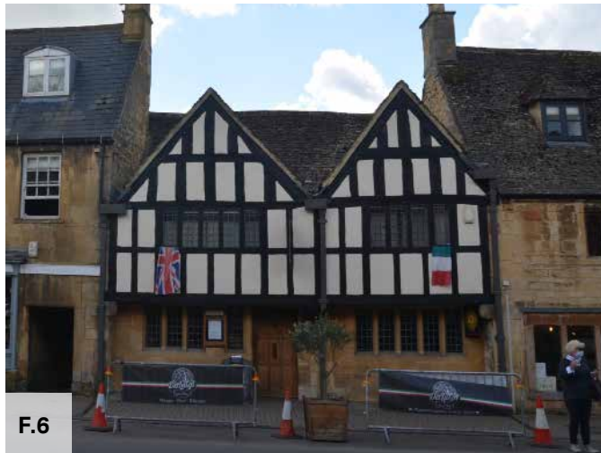
Figure 06: Timber framing, High Street
