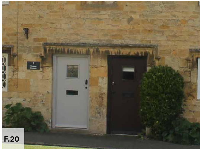
Figure 20: Ashlar dressings, Leysbourne
