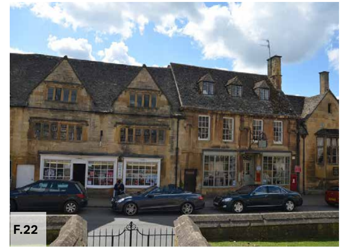
Figure 22: Stone slate roofs, High Street
