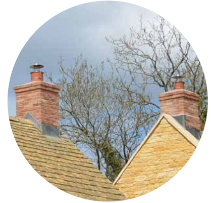
Red brick chimneys
