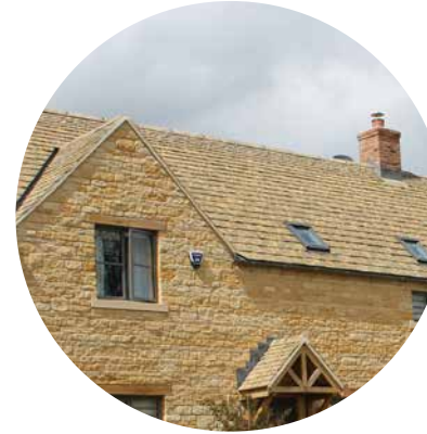
Local stone in irregular courses, stone slate roof in diminishing courses, brick stacks
