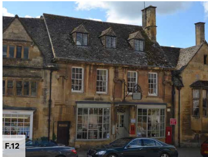
Figure 12: The Post Office, High Street
