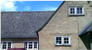
Showing the whoosh at the base of a modern tiled roof
