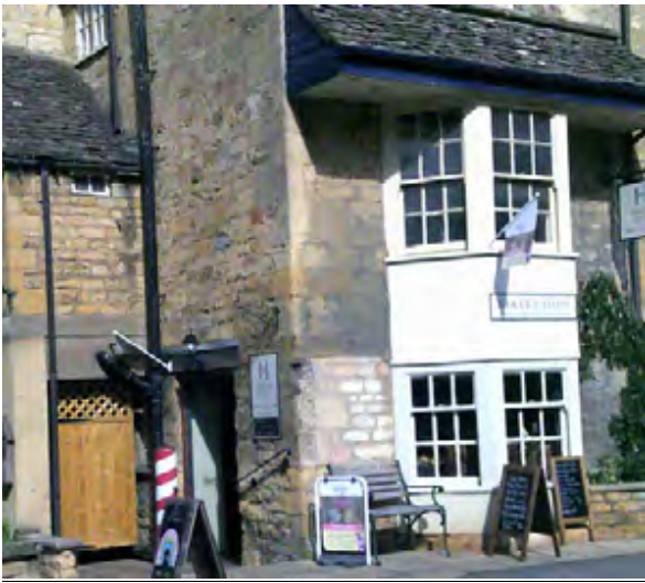
Before demolition High Street
