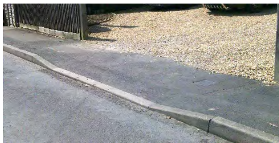
one lowered kerb leaves parking for visitors or delivery vans on highway without reducing the cars parked on site.
