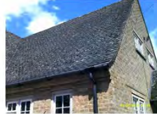
Showing the whoosh at the base of a modern tiled roof
