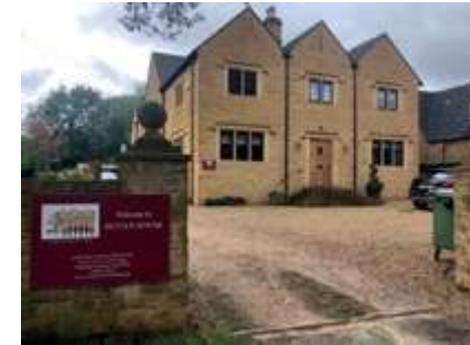
Jecca's House (Campden Home Nursing) Jecca's House, Aston Road, Chipping Campden, GL55 6HR
