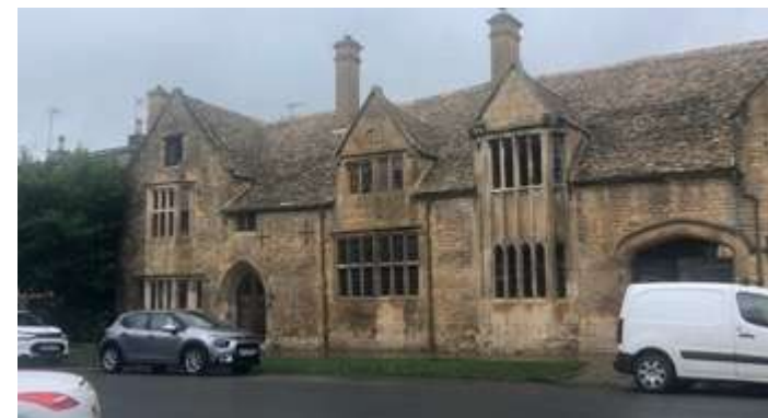
Figure 12: Grevel House; 14th Century, Grade I listed.
