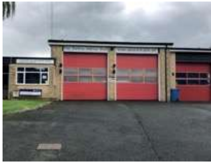
Community Fire & Rescue Station Catbrook, Chipping Campden, GL55 6DG
