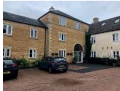
Mill House Care Home 55 Sheep Street, Chipping Campden, GL55 6DR
