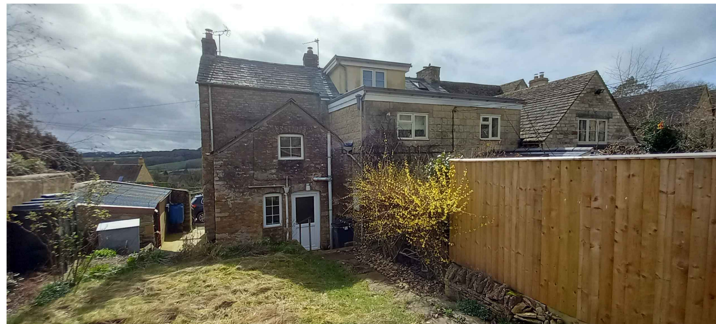
VALLEY VIEW - REAR PHOTOGRAPH
