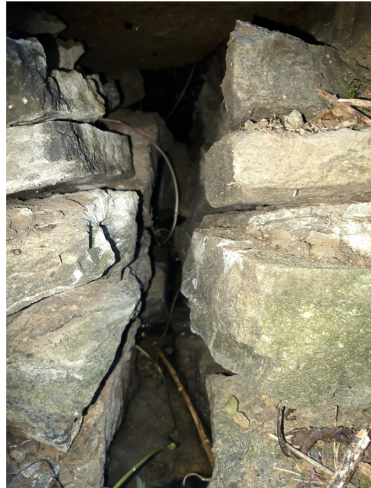
Photograph 12 – Inside the dry-stone outfall
