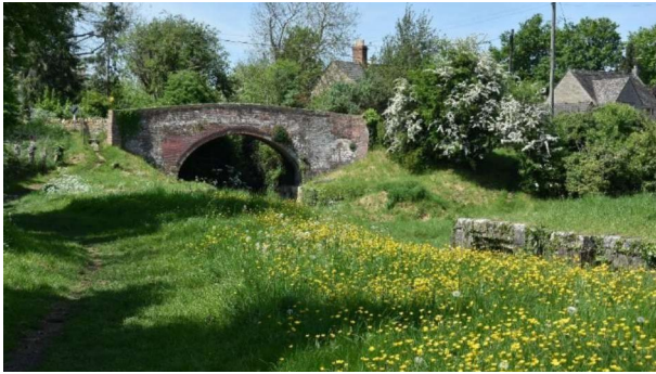
Figure 61 Upper Siddington Bridge
