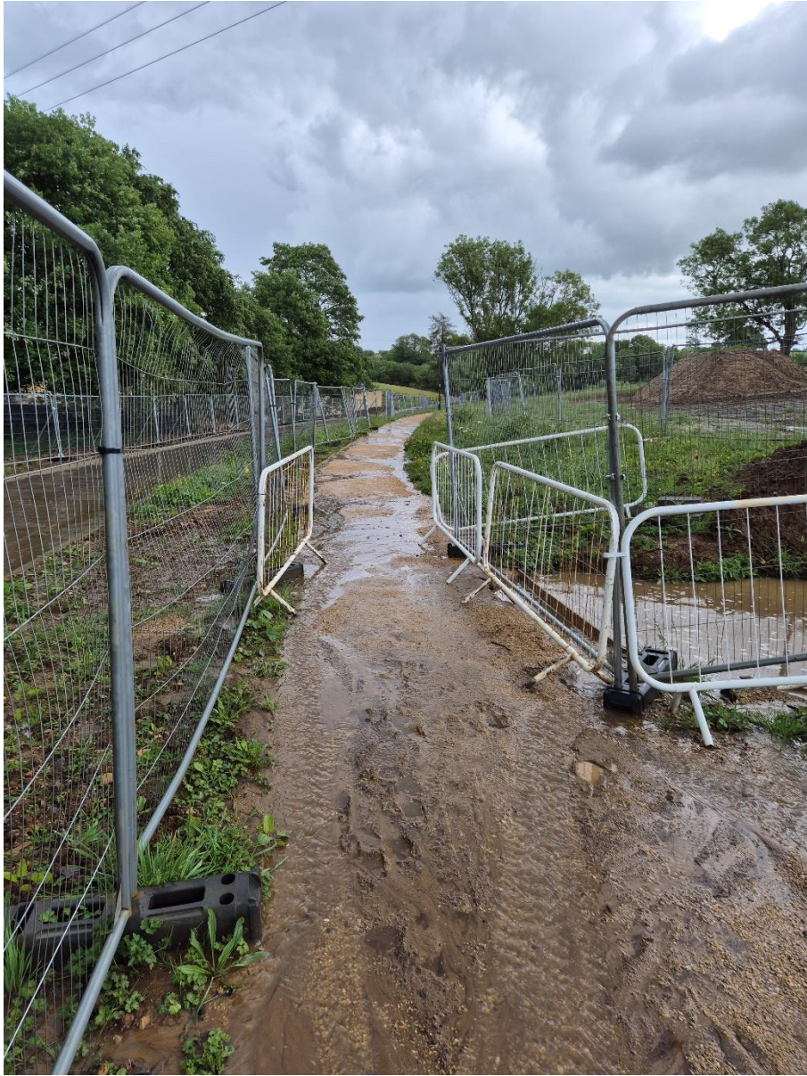
New path as constructed (1)
