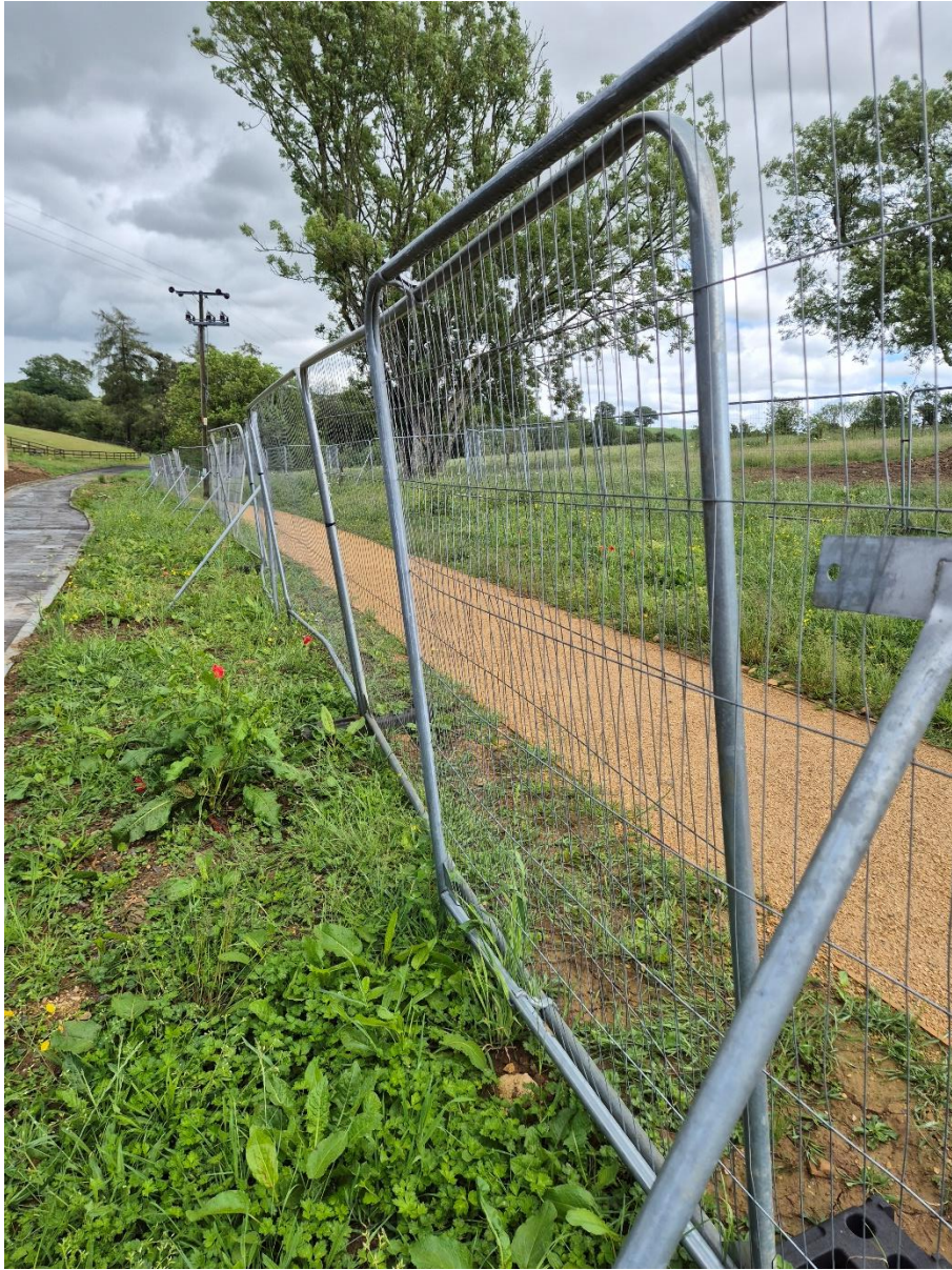
New path as constructed (2)
