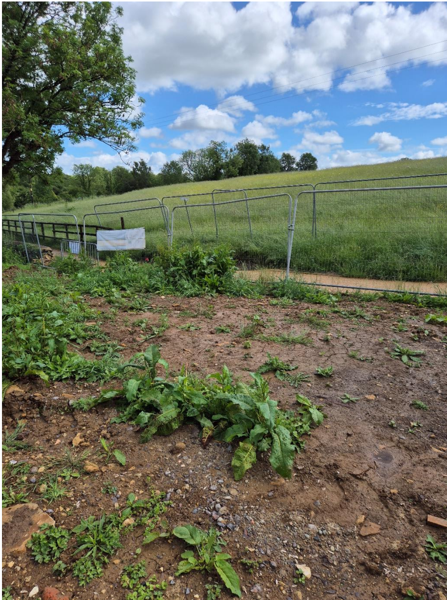
Path as constructed linking to existing public right of way
