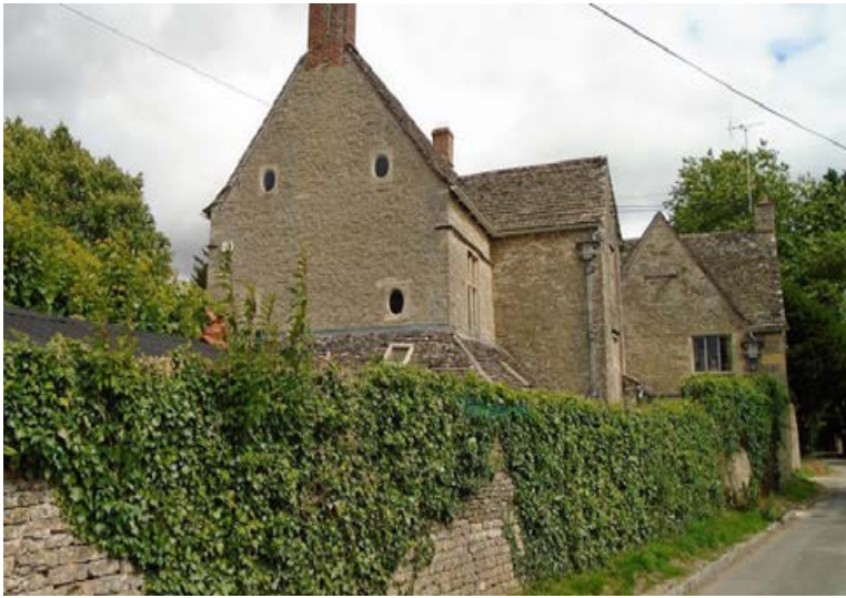
Figure 49 Roberts House. View 6C
