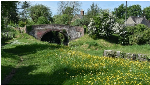
Figure 61 Upper Siddington Bridge
