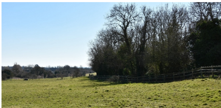
Figure 36 View of St Peter's Church from meadow next to Siddington Road. View 3B
