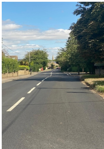
Figure 37 Ashton Road through the village from the south. View 4A
