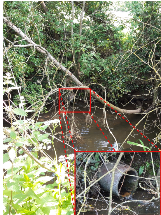
Photograph 10 – Highway drain outfall into Poulton Brook
