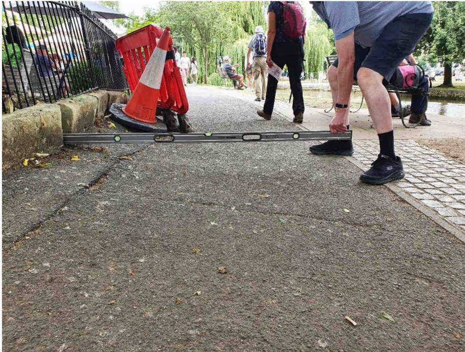
Photograph 5 and 6. Vertical displacement of footpath and developing radial cracks
