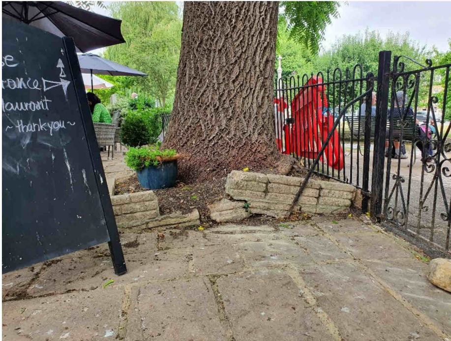
Photograph 7. Displacement of internal retaining wall and paving.
