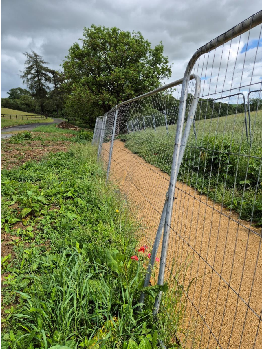
New path as constructed (3)
