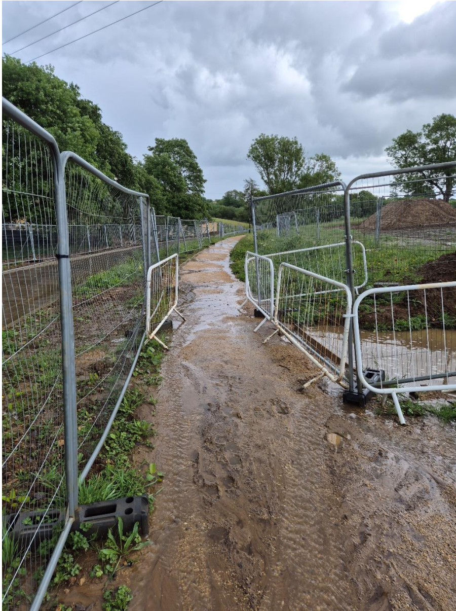
New path as constructed (1)
