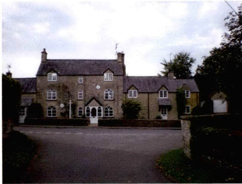
Figure 17: An unlisted cottage, with a blue slate roof, and distinctive arch-headed windows.
