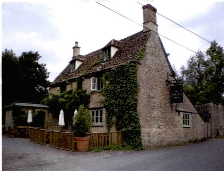
Figure 14: The Bakers Arms pub (Grade II Listed) dates to the eighteenth century.
