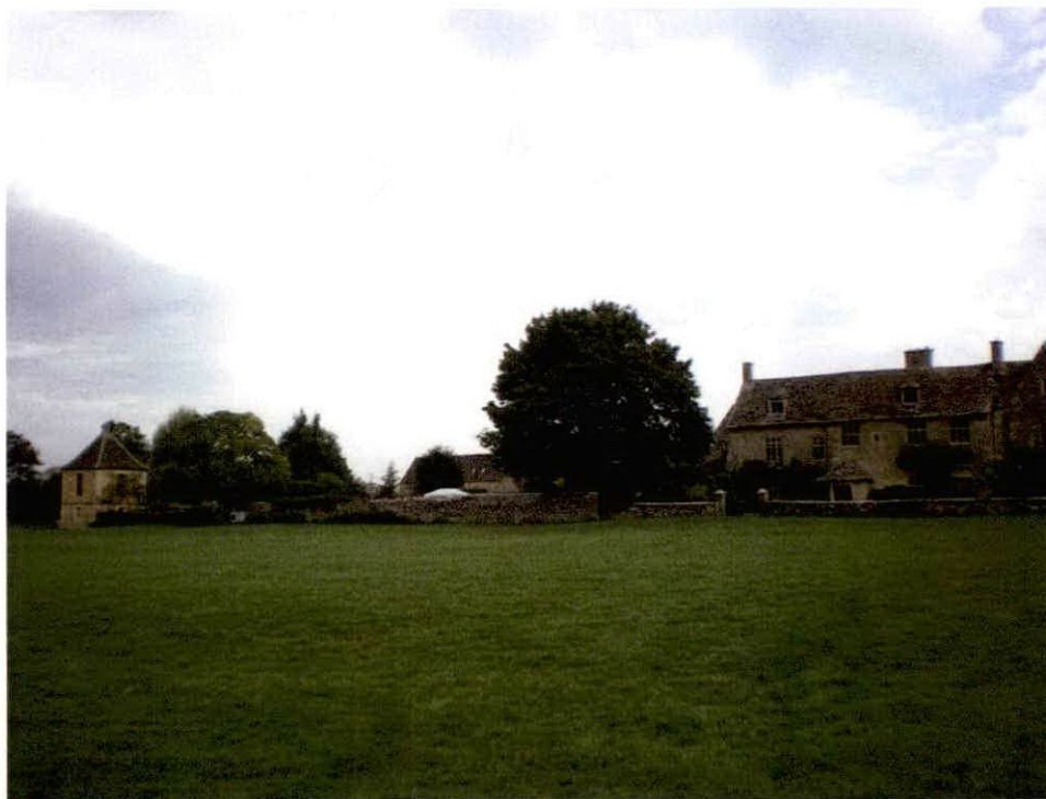
Figure 7: The Manor House is Grade II Listed and dates to at least the sixteenth century, but it is largely seventeenth century. It is typical of a higher status Cotswold vernacular house of that period, with stone tiled roof, large gables, stone cross-mullioned windows and Tudor-arched doorways. To the west there are further listed farm buildings relating to the Manor.
