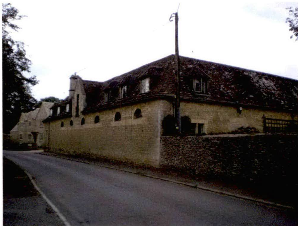
Figure 11: The large stable block (Grade II Listed) adjacent to the Dower House, built in about 1920, has a plain clay tiled roof, with hipped dormers, and high level half-round windows set within stone surrounds.
