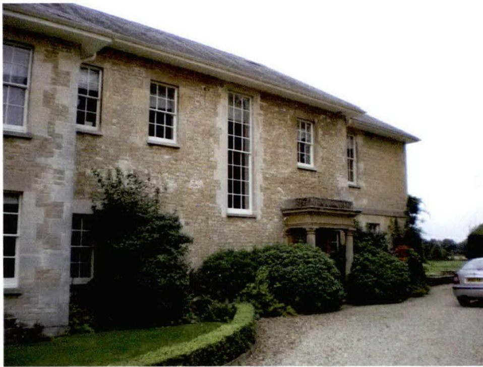
Figure 9: Somerford Keynes House (Grade II Listed) dates to 1804 and is a large house built in the classical style, with overhanging hipped slate roof, sash windows and a Doric porch. The house is set within attractive grounds, open to the former parkland to its west.
