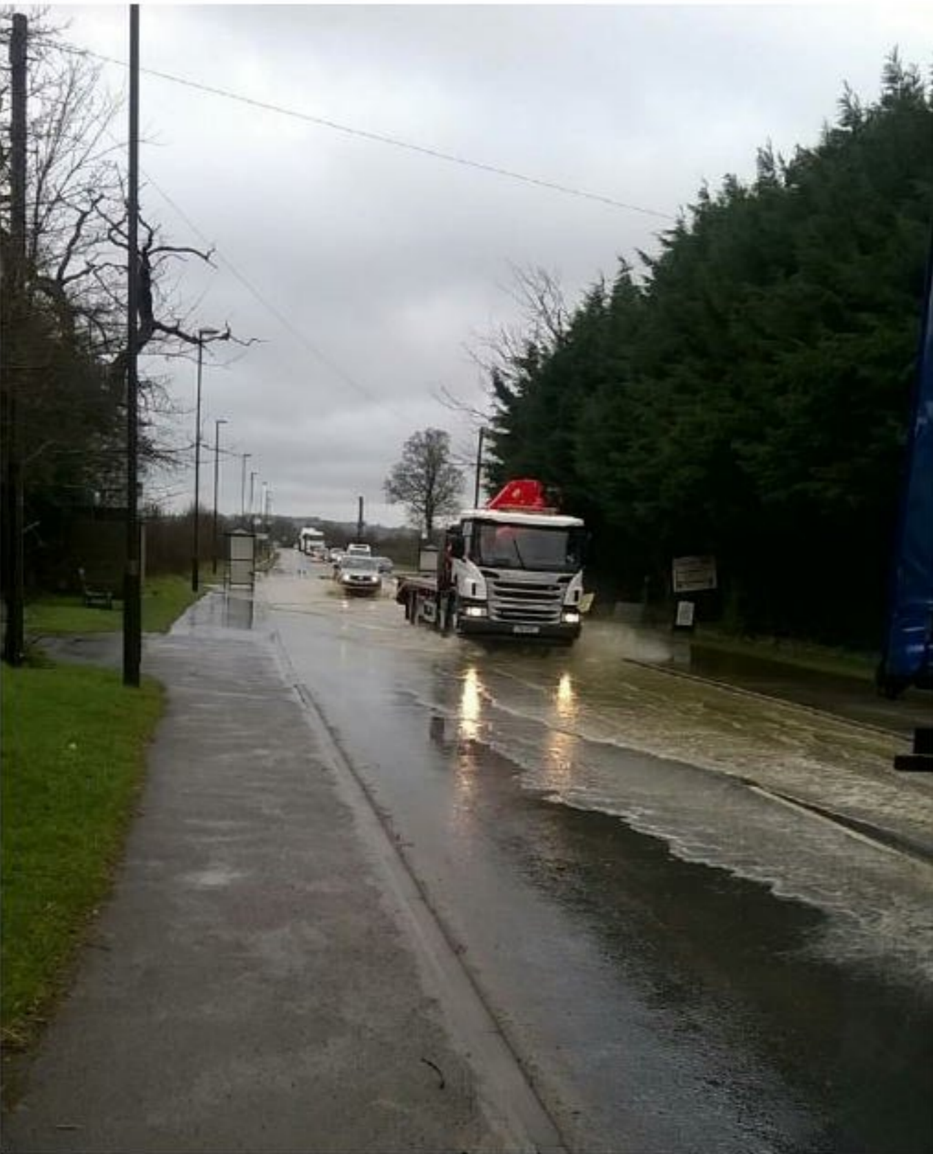
9/3/2016 flooding across the A429 where Aldi is now.
