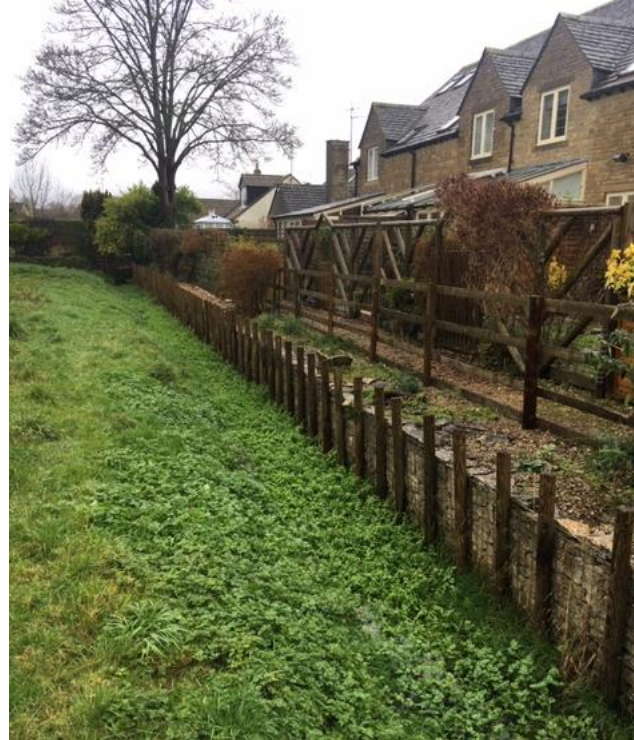
Figure 2 Drainage ditch 12th December 2019 (wettest December on record)
