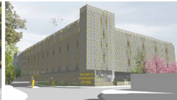
View of vehicular entrance
